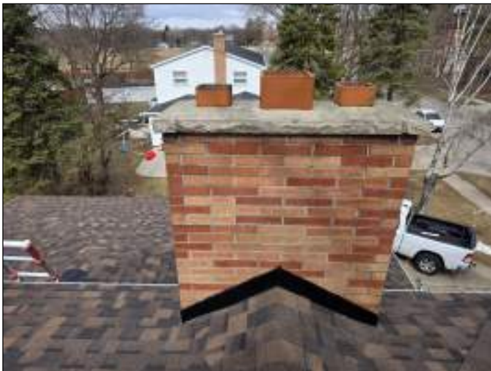
Example photos of the chimney.
