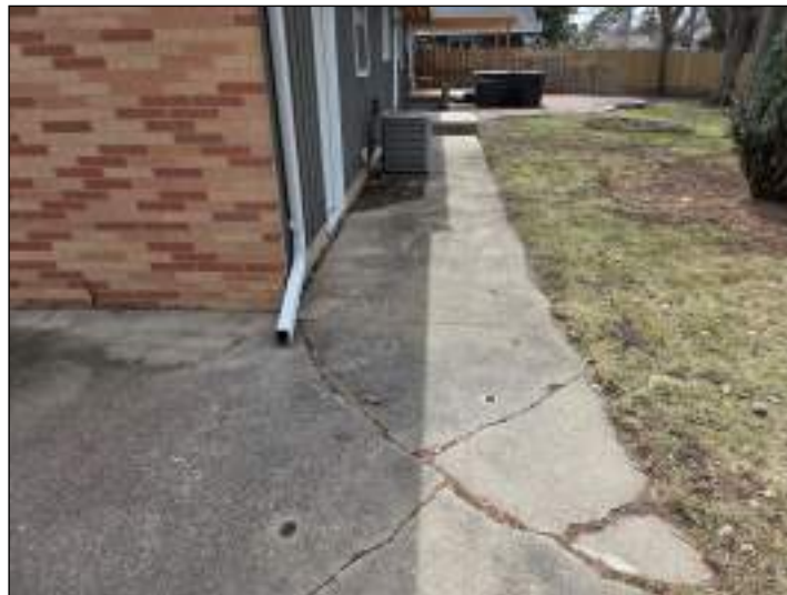
The slabs in front of the garage door opening settled.
