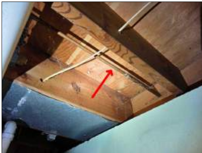
I recommend adding a shut-off valve in the basement.
