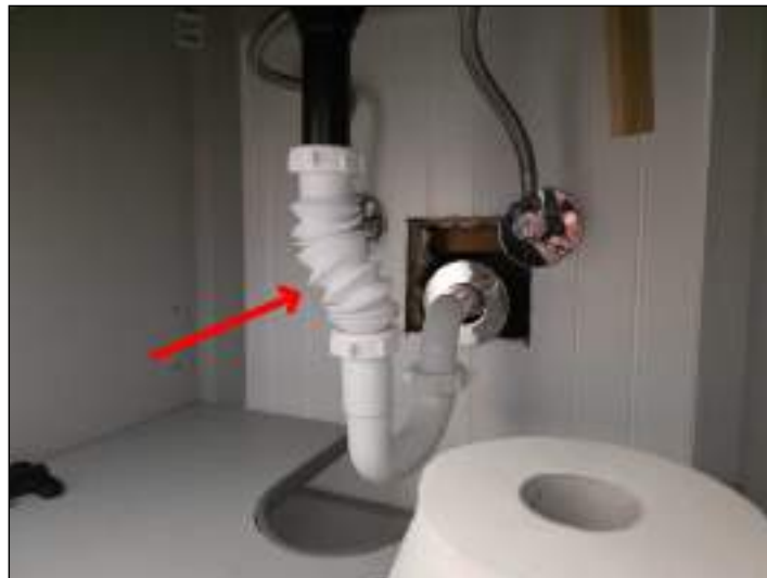
Corrugated / flexible piping was installed.
