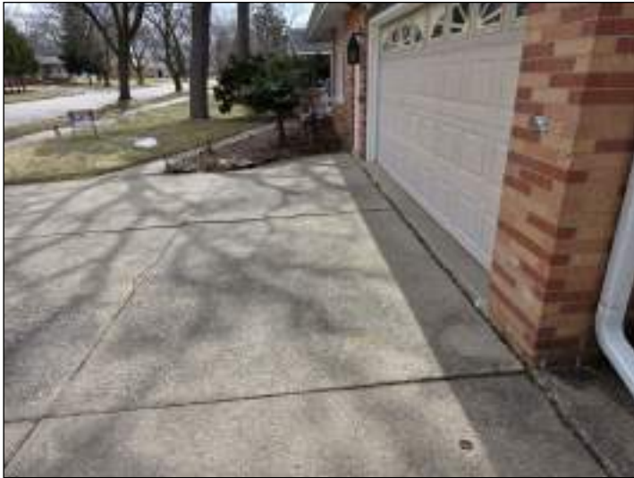
The slabs in front of the garage door opening settled.
