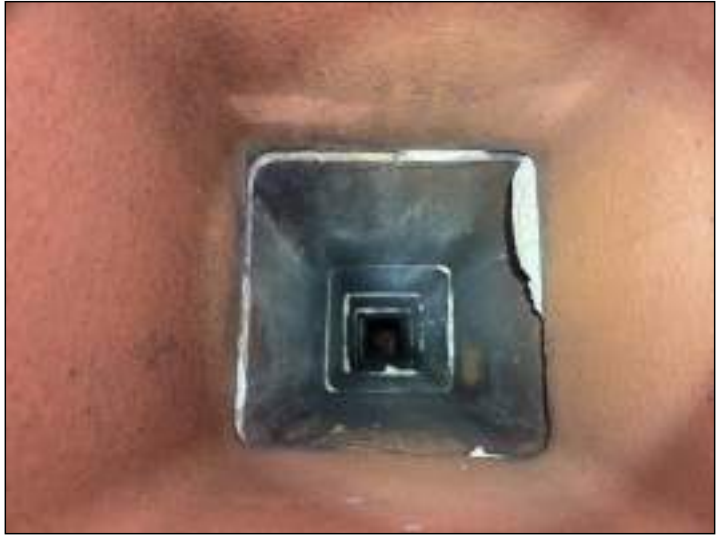
View down the flue for the fireplace.
