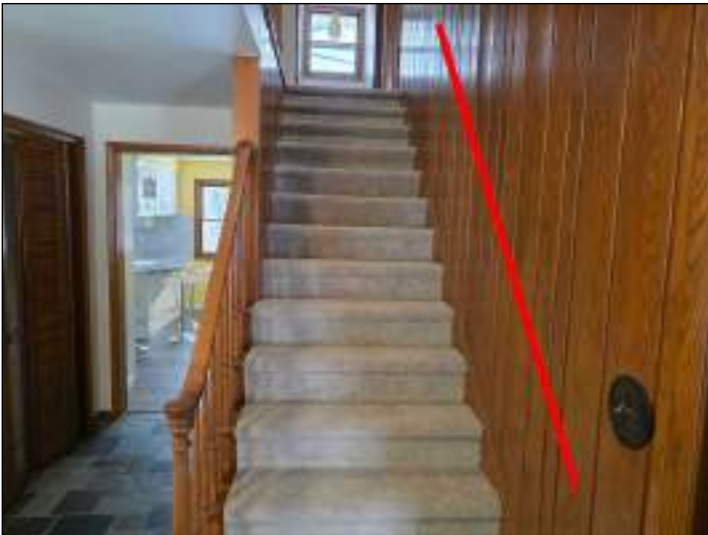
I recommend adding a continuous handrail on this stairway.
